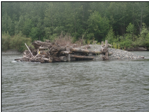
Logjams restore habitat for juvenile salmon on the Nooksack River. Photo Credit: Oliver Grah
